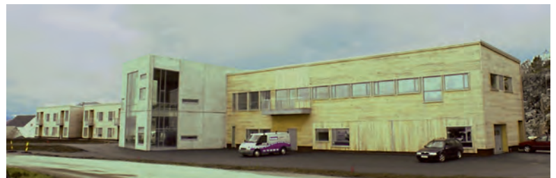
Fig. 1: The building of the Runde Environmental Centre, Norway
